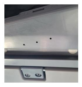
• Drill through the three marks with a 3/16 inch drill bit.
